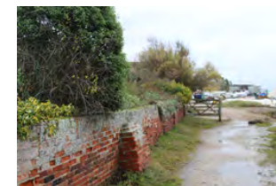
Figure 60 Example of historic walls
