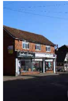
Figure 75 Modern Shop Front
