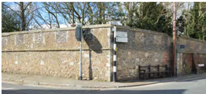
Figure 30 Stone section of wall
