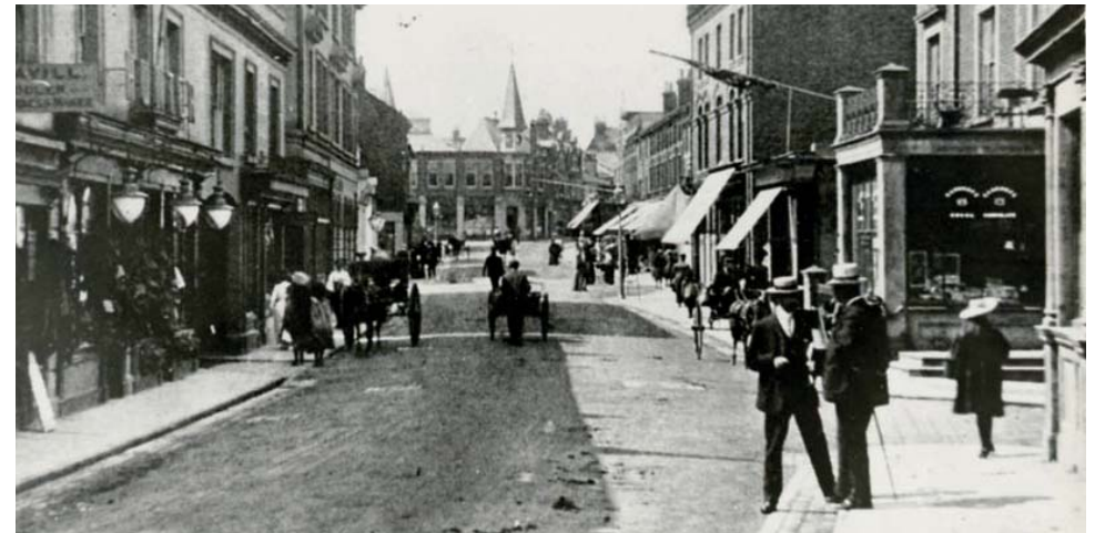
Figure 43 Scoria bricks visible lining the gutters along the High Street (1920)
