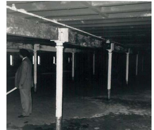
Figure 12 A photograph taken in 1991, showing the interior of the maltings, with cast iron columns, a floor surface of setts and timber structure of the first floor (Essex County Council)
