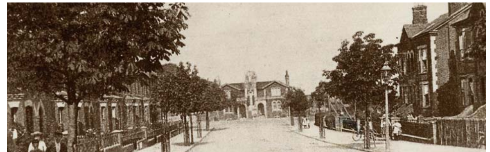
Figure 44 Trees along Station Road, 1910
