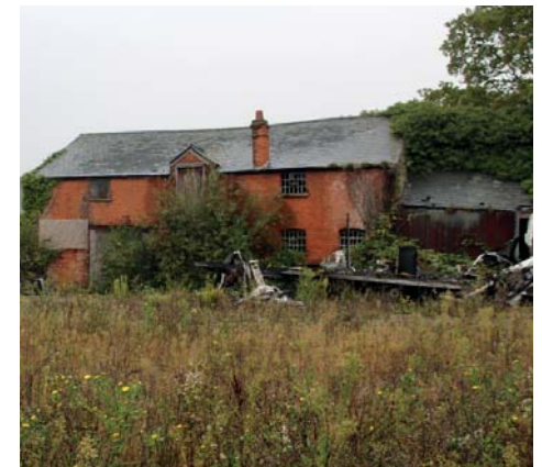
Figure 16 The stables and coach house of the King Edward Public House
