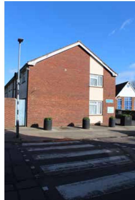
Figure 87 Unsympathetic street lighting
