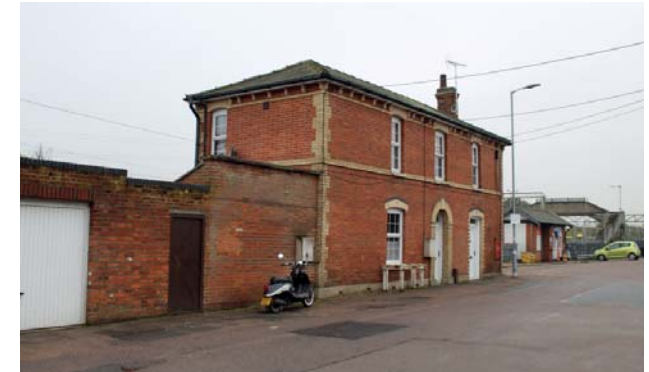
Figure 18 A photograph of the station master's building today after refurbishment and reuse as two residential properties
