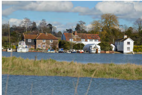
Figure 65 Gambrel roof Summer Cottage
