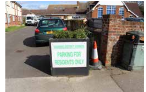
Figure 88 Signage and bin in poor condition
