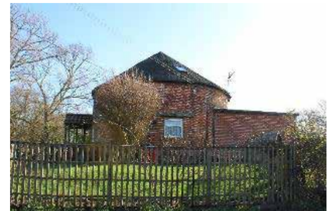
Figure 33 Remains of Old Mill
