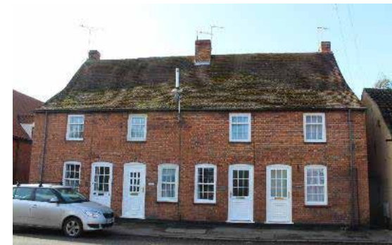
Figure 77 Unsympathetic Additions - satellite dishes
