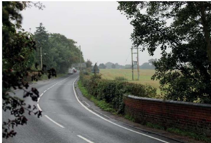
Figure 44 Rice Bridge and the open rural landscape to the south of the Conservation Area
