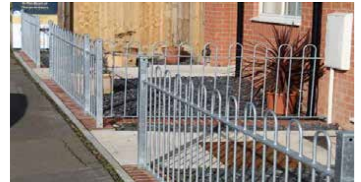
Figure 51 Steel railings outside a recent development on the High Street have a detrimental impact on the character of the Conservation Area
