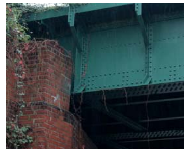
Figure 22 A detail of the railway bridge
