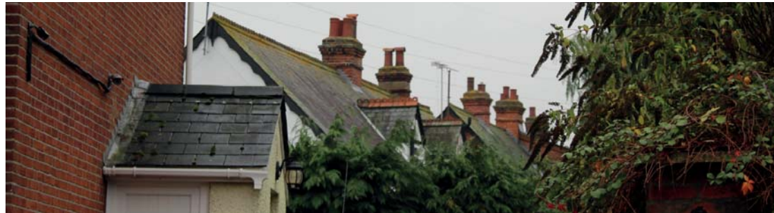
Figure 30 A glimpsed view of the chimneys of the Edward Road buildings
