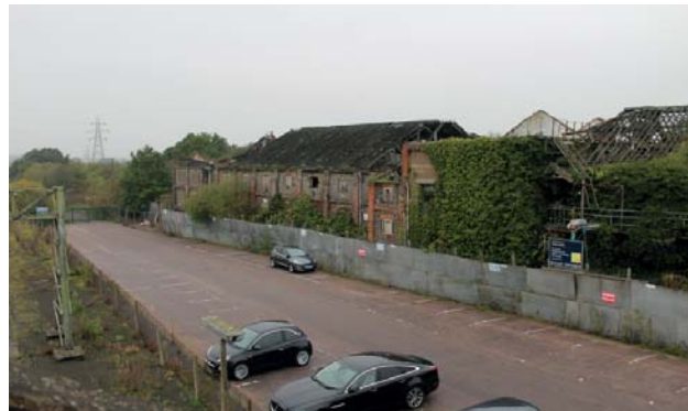
Figure 39 Viewpoint 2 looking north-west
