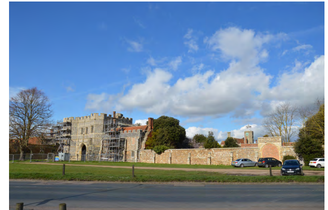
Figure 71 Flushwork of the Priory gatehouse
