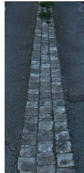
Figure 35 Scoria bricks on Crown Lane
