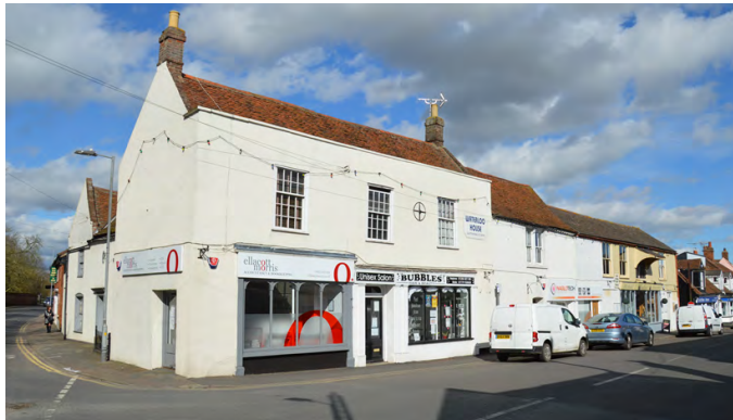
Figure 35 Commercial units and residential properties located close the junction of Clacton and Spring Road
