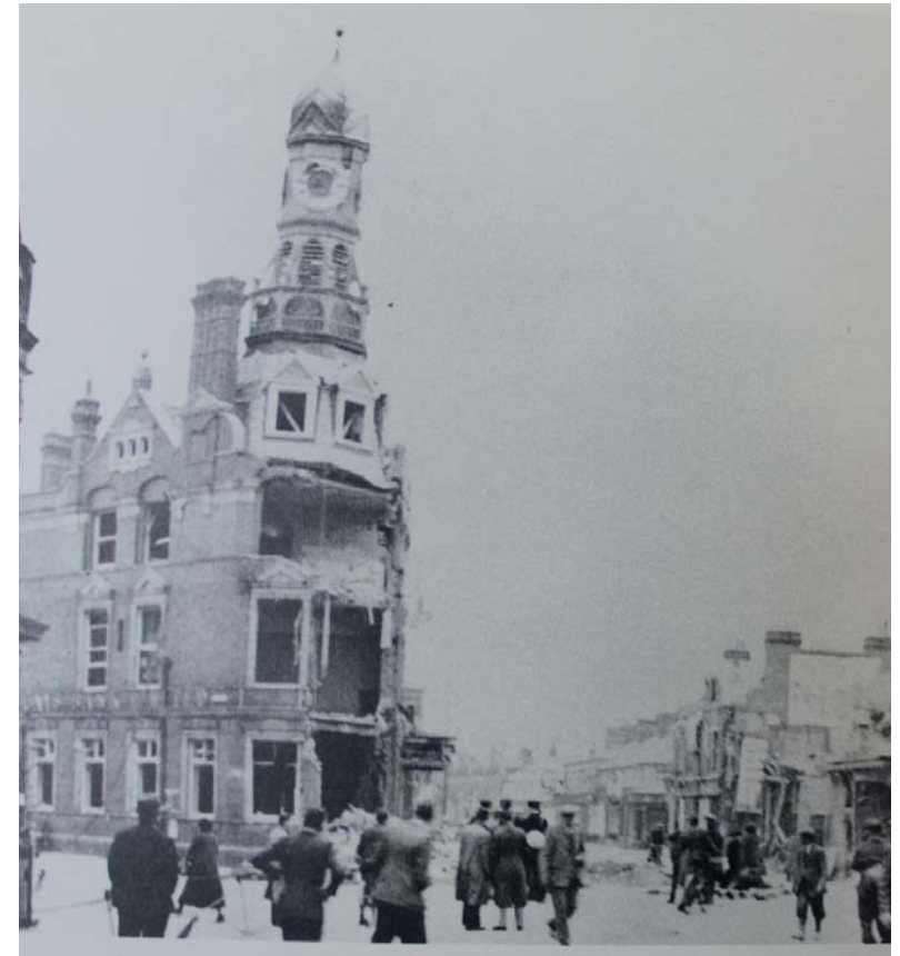
Figure 12 Air Raid Damage 1941 (Britain in Old Photographs 1995)
