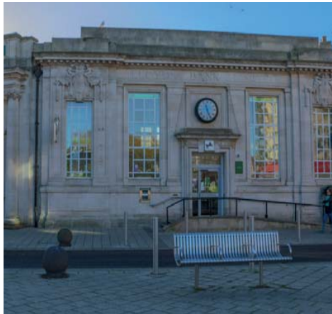
Figure 24 Lloyds Bank Building
