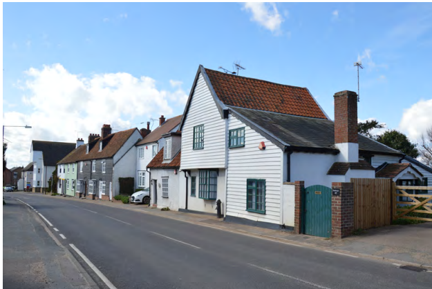
Figure 61 Numbers 45-49 Mill Street
