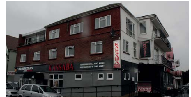
Figure 18 Example of inappropriate signage and paint colour on West Marine Parade
