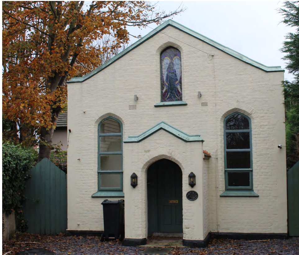
Figure 31 The Old Chapel 30 Colchester Road
