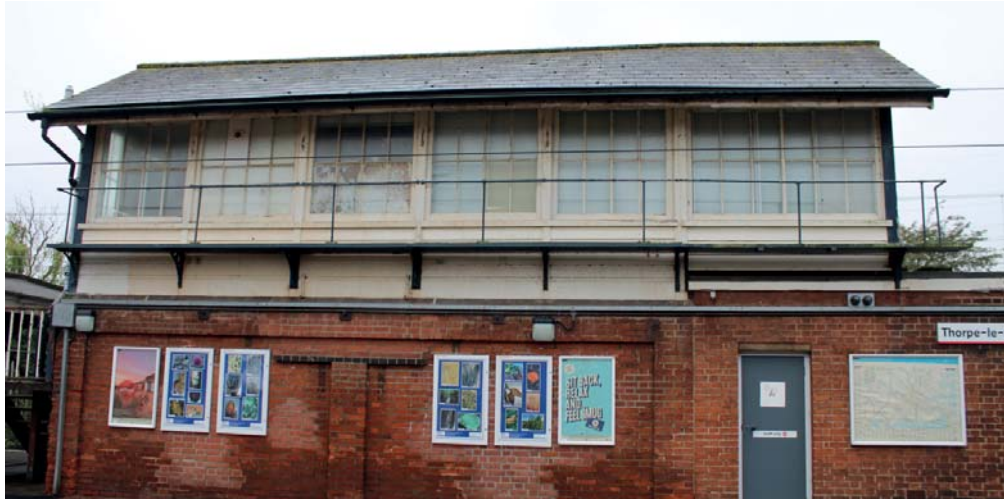
Figure 20 The signal box on Thorpe-le-Soken's island platform
