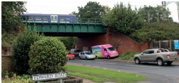
Figure 21 Thorpe-le-Soken railway bridge
