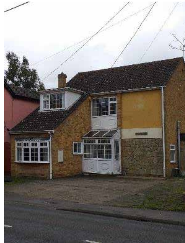
Figure 86 Modern development that does not reflect form, design or material of the Conservation Area
