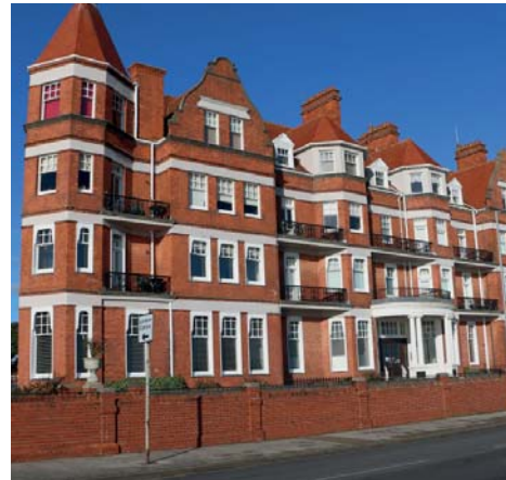
Figure 34 Colchester Institute (Grade II Listed)
